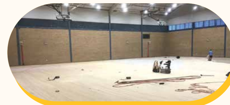
Slipping and sliding is minimal on the upstairs multi-purpose courts at SUSAC after they were sanded and refurbished over the break with members providing very positive feedback since their return.
