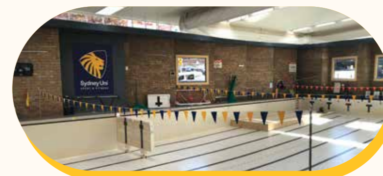
It took a total of five weeks to provide essential maintenance works to the pool in the plant room – a project that was sitting on SUSF's to-do list with draining needed in order to go ahead.
